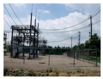
Figure 4.14. An Open-Air Substation (Note: Absence of Secondary Containment)
