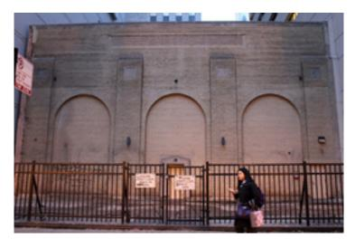
Figure 4.13. An Enclosed Substation (Note: Indoor Design Blends in with its Surroundings)
